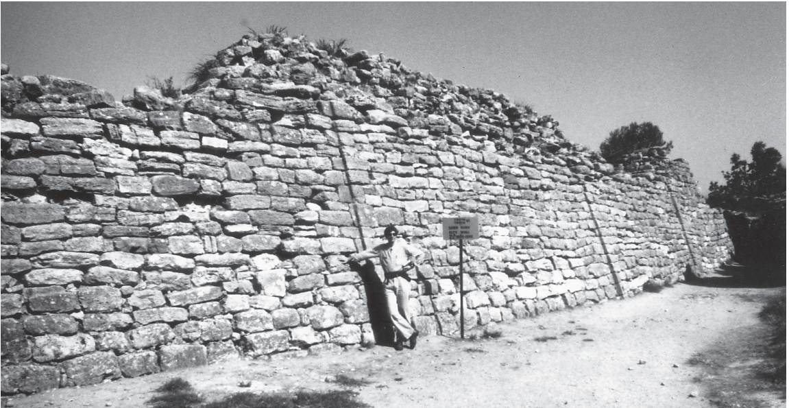
FIGURE 1.2 The author at the walls of Troy. The earliest settlement at Troy can be dated to about 3000 BC, but the citadel walls shown here belong to the sixth level of occupation (Troy VI), built around 1400 BC and destroyed around 1230 BC. Constructed of neatly cut blocks of limestone that slope inward, the citadel wall had at least four gateways, two of them protected by towers. Either Troy VI or its much poorer successor Troy VIIa, destroyed about 1180 BC, could have inspired Greek legends of the Trojan War. (Author's photo)
